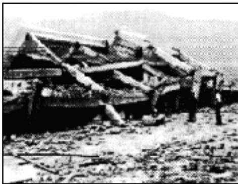
Officials inspecting ruins of school building in Cangyuan province, China
