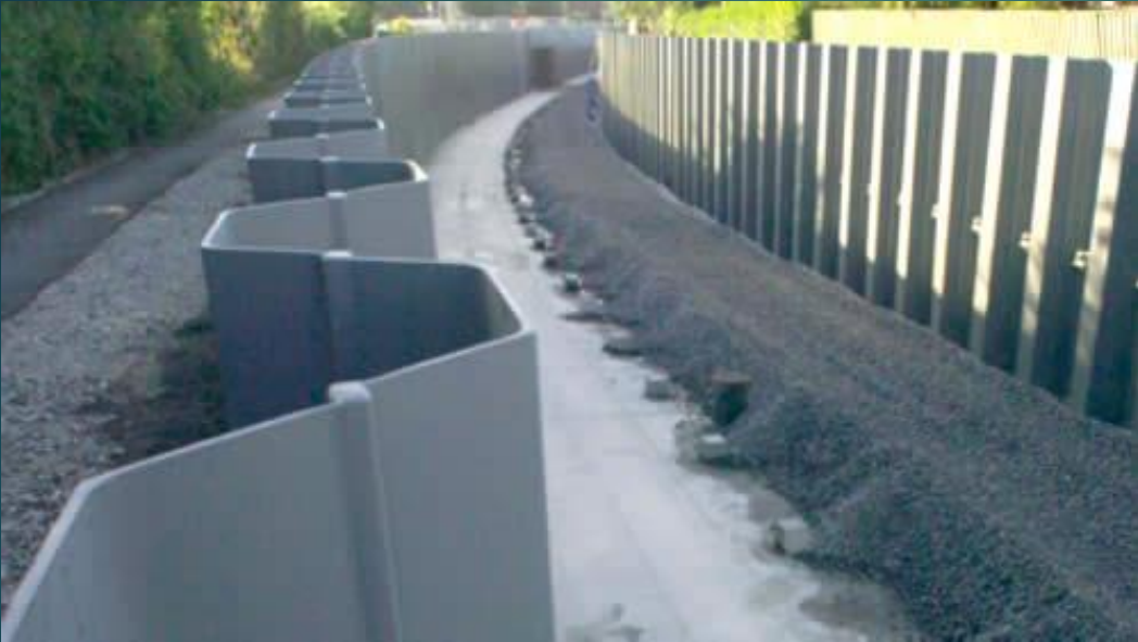
SHEET PILE CUTOFF WALL
