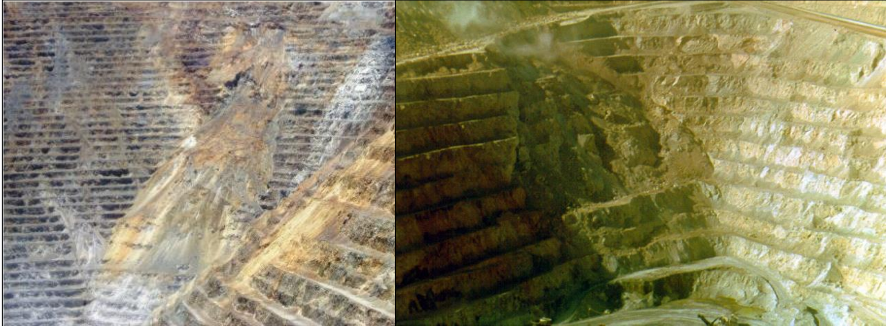
Bingham Canyon mine slope failure
