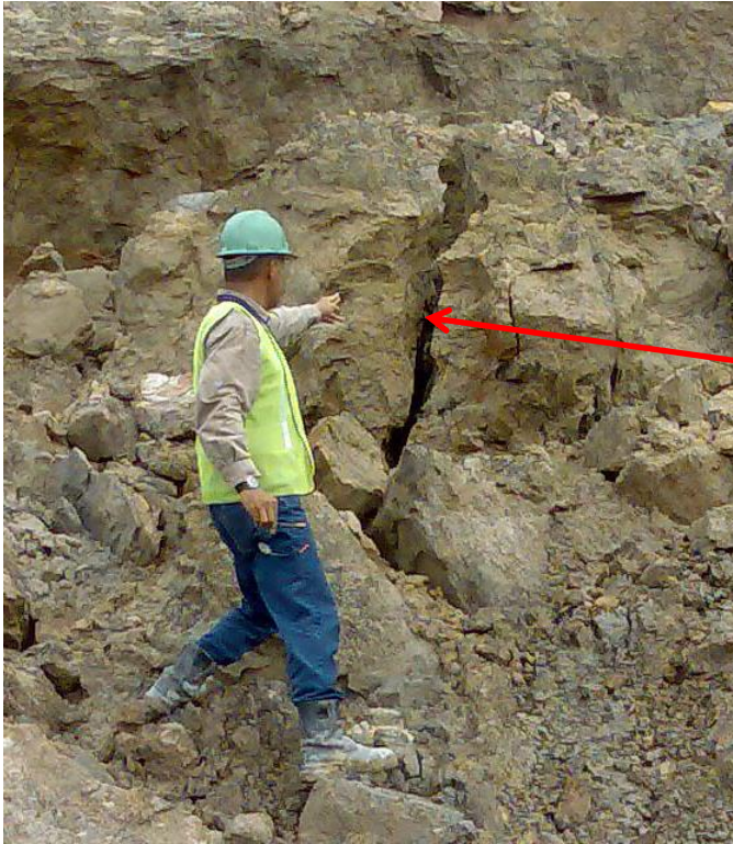
Individual slope rock mass failure due to joint and weather factors.
